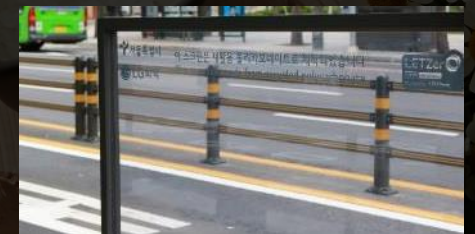
Bus stop built with PCR materials
