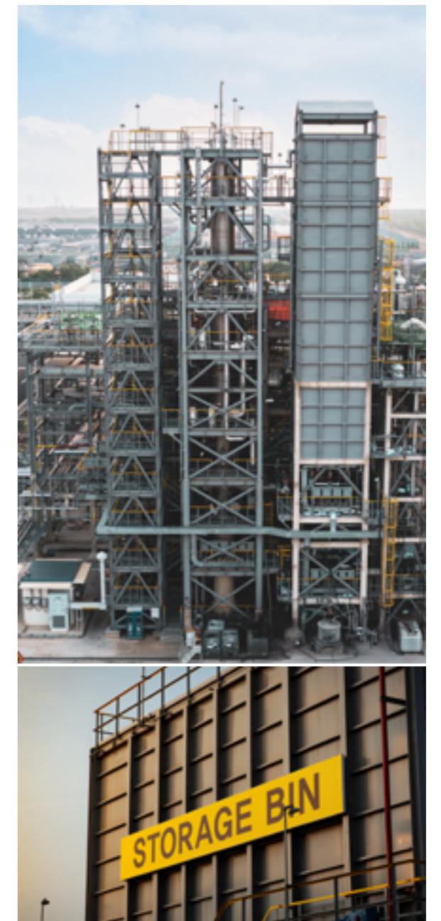
LG Chem Dangjin Chemical Recycling Plant
